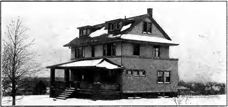
Private residence, leased by National Lamp Works, used by Purchase, Contract, and Transportation Sections, Development Division.
